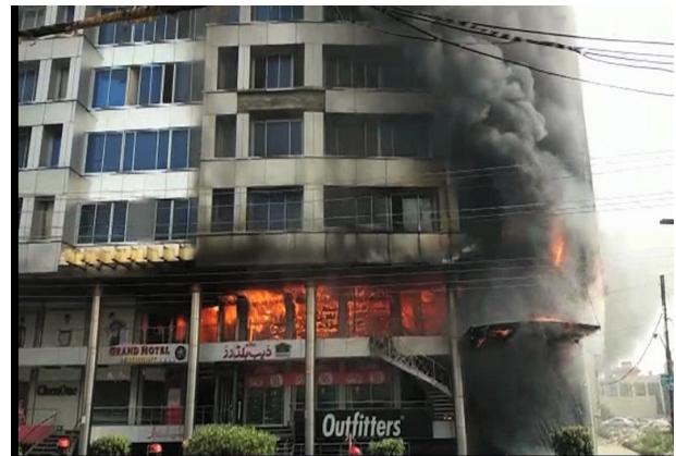
Fire incident at Alina Center, Gujrat (2019)
