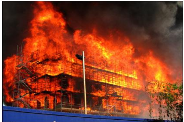
Fire incident at Lahori Gate, Lahore – Jan 2016
