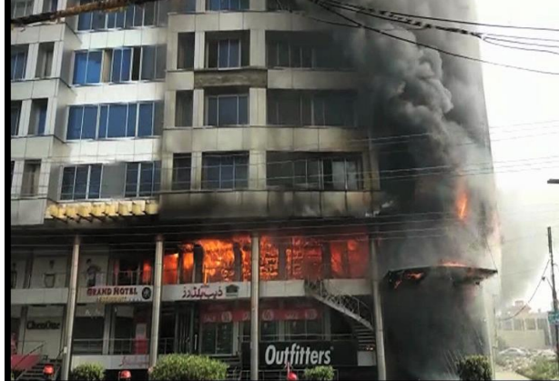
Fire incident at Alina Center, Gujrat (2019)
