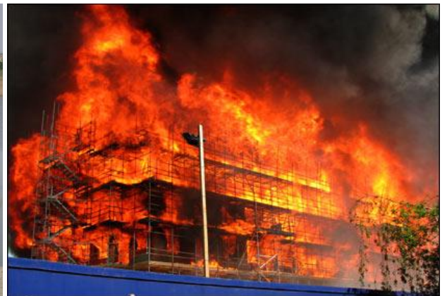
Fire incident at Lahori Gate, Lahore – Jan 2016
