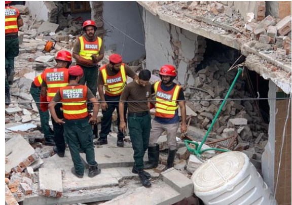
Building Collapse (Gujrat - 2021)
