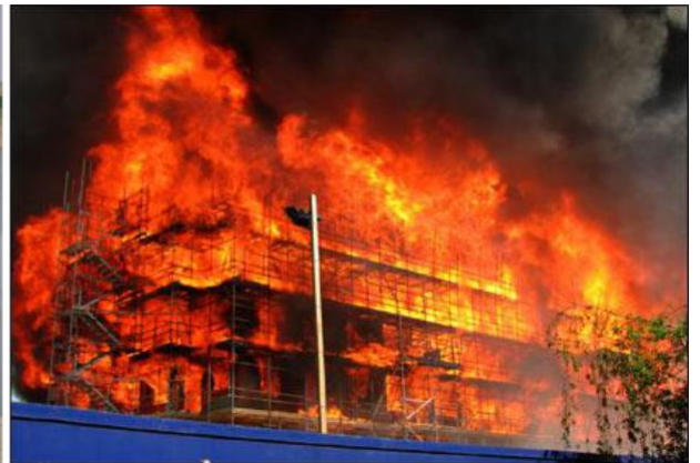
Fire incident at Lahori Gate, Lahore – Jan 2016
