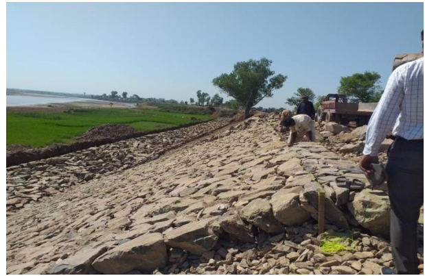
Jalala Flood Protection Bund.
