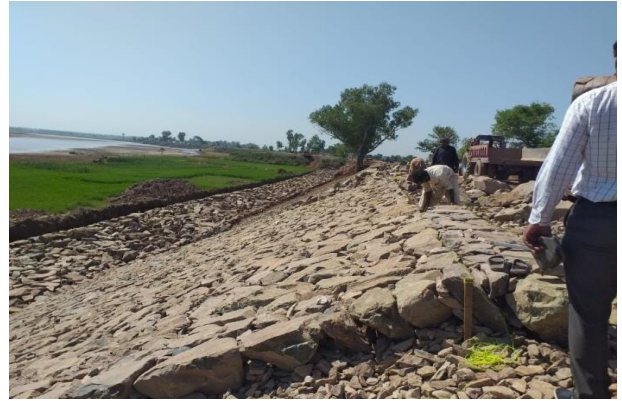
Jalala Flood Protection Bund.
