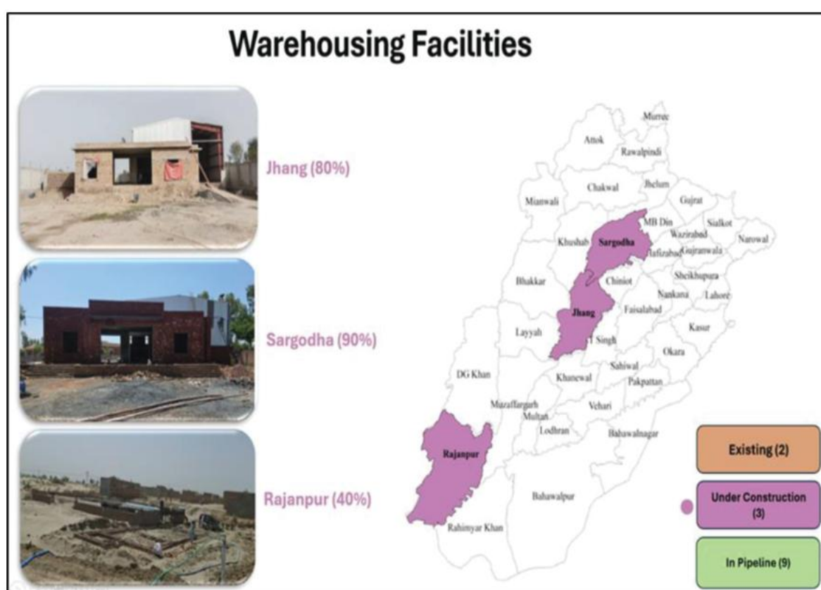
Figure 49: Status of Completion of Warehousing Facilities
